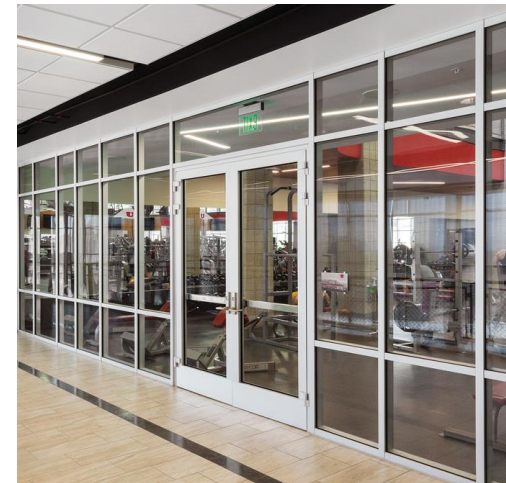
4 Storefront: Aluminum and Glass door and partitions
